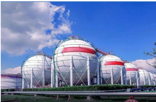
oil depot and chemical tank area
