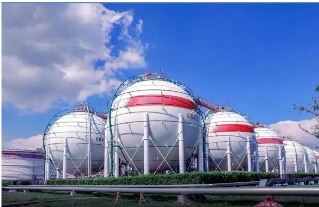
oil depot and chemical tank area
